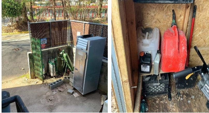
**Photograph 10 (left): Oxygen cylinders stored in unsafe manner, not protected from weather.**
