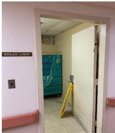
**Photograph 8 (left): Door to laundry chute room containing combustible materials propped open.**
