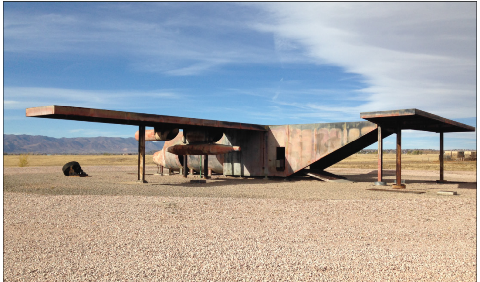
Figure 3: Current Fire Training Area at Peterson Air Force Base, Colorado
