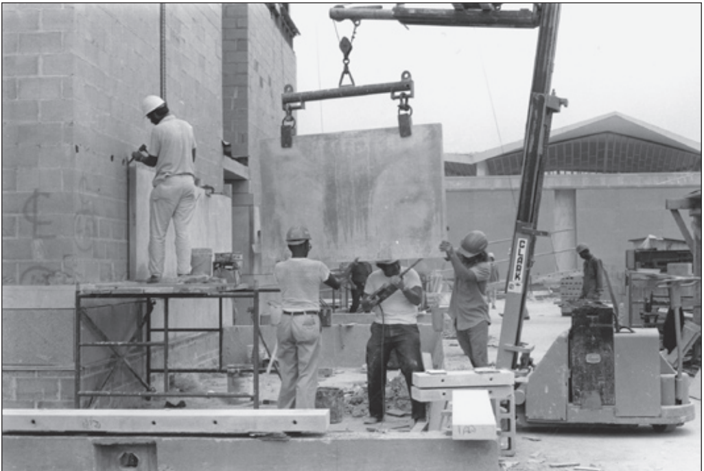
Above is a view of the construction of the library's Lister Hill National Center for Biomedical Communications looking south toward Bethesda in late 1978. This area would eventually become the location of the parking deck for the center. The view below from mid-1979 looks east as workers install portions of the limestone facade, with the original library building in the background.
