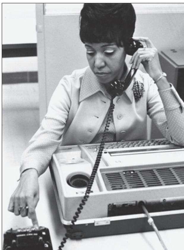
Librarians Gerry Nowak (above) and Yvonne Scott (right) use acoustic couplers (early computer modems) to establish a connection to a mainframe computer, which enabled access to MEDLINE in the mid-1970s.
