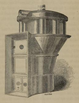
This Furnace is constructed with an iron base and ash pit, similarly to several others. It has a recess front, connecting the ash-pit and feeding apparatus, with large doors for removing the ashes and cinders, and for putting in the fuel. The front is so attached to the base and mouth-piece that it can
