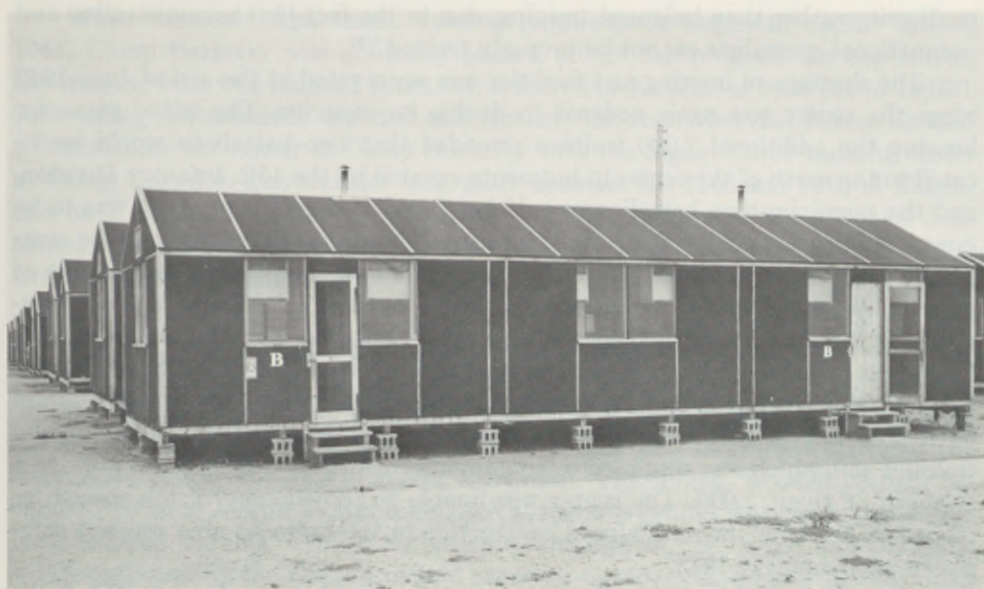
FIGURE 23.—Hutments used to house trainees at Camp Barkeley, Tex.
