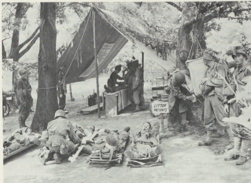
FIGURE 25.—Trainees set up and operate an aid station as part of their tactical training at Camp Grant, Ill.
