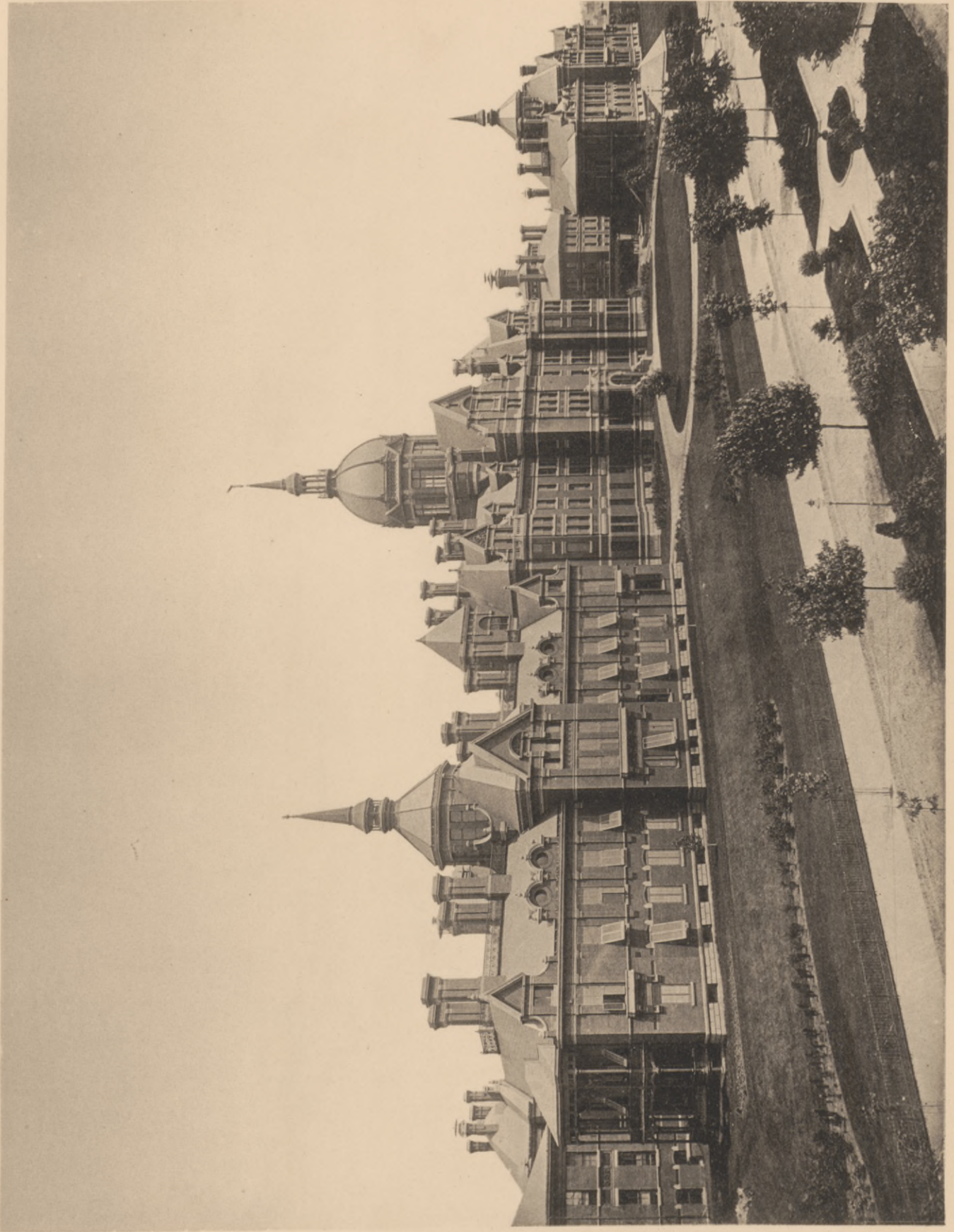
FRONT VIEW OF BUILDINGS FROM NORTHEAST.
