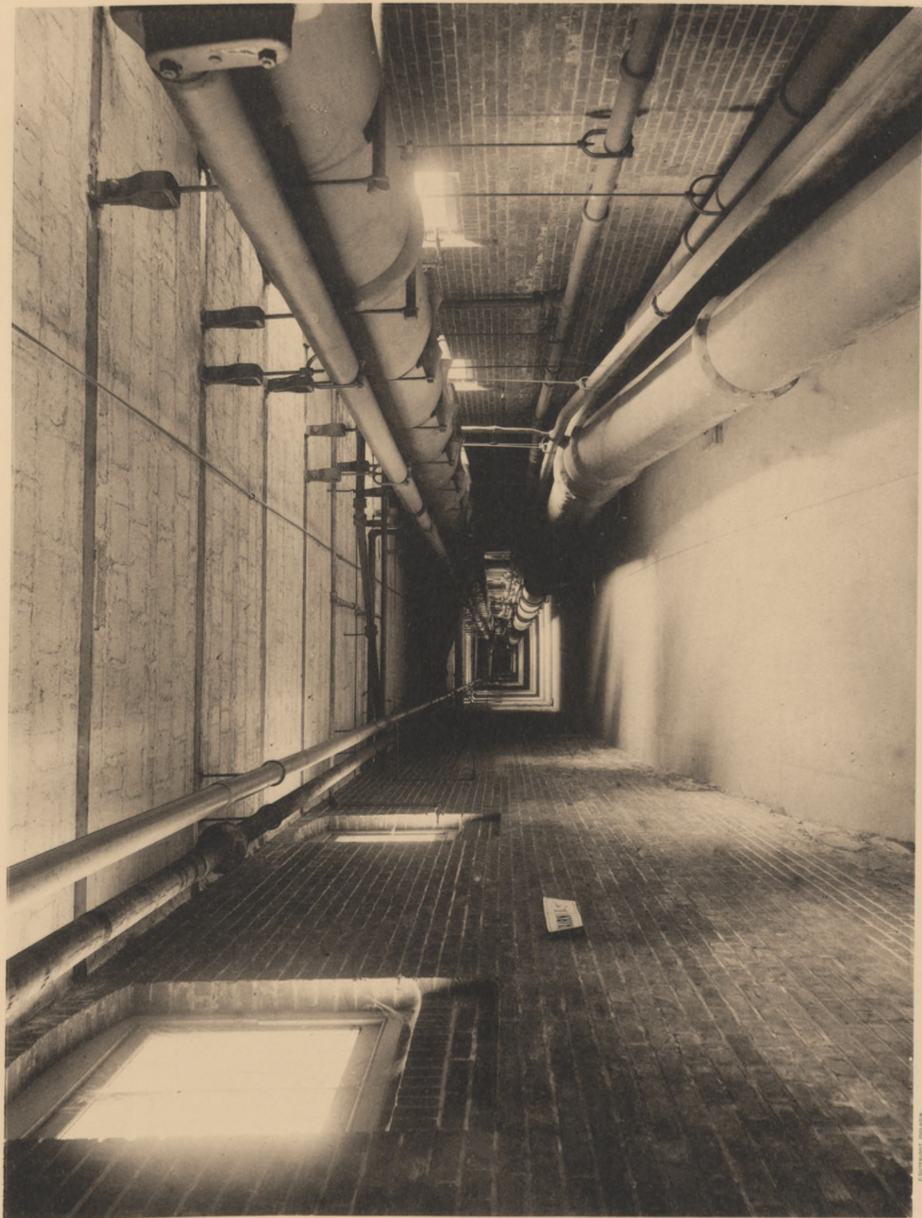
PIPE TUNNEL INTERIOR VIEW, LOOKING EAST.
