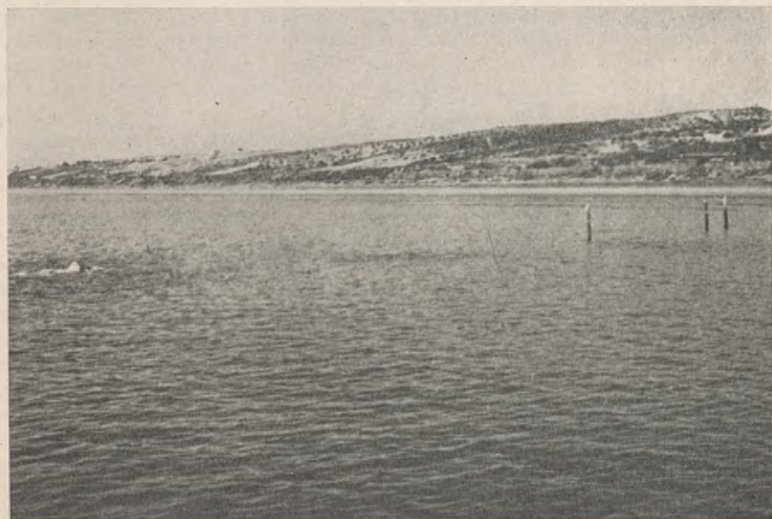
FIG. 5. Leak in Submarine Outfall thought to be due to manhole blowing off in October, 1942, is shown at left of photo. Note other leaks to the right of this one.
