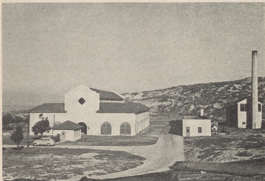
FIG. 2. Outside of Main Fine Screening Plant at Hyperion.
