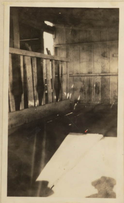
Interior of Milking Shed at Private Dairy
