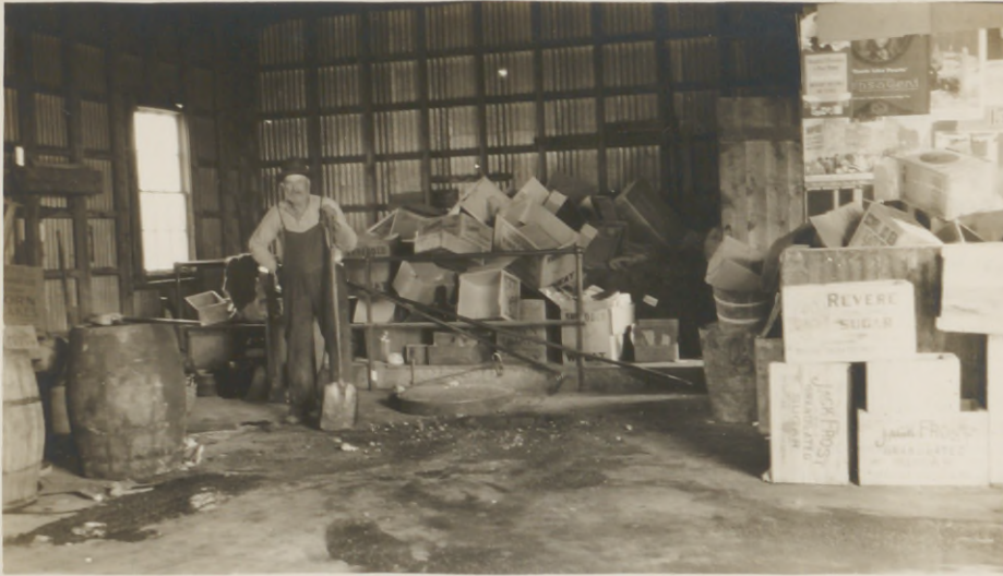
Interior of Incinerator Plant
