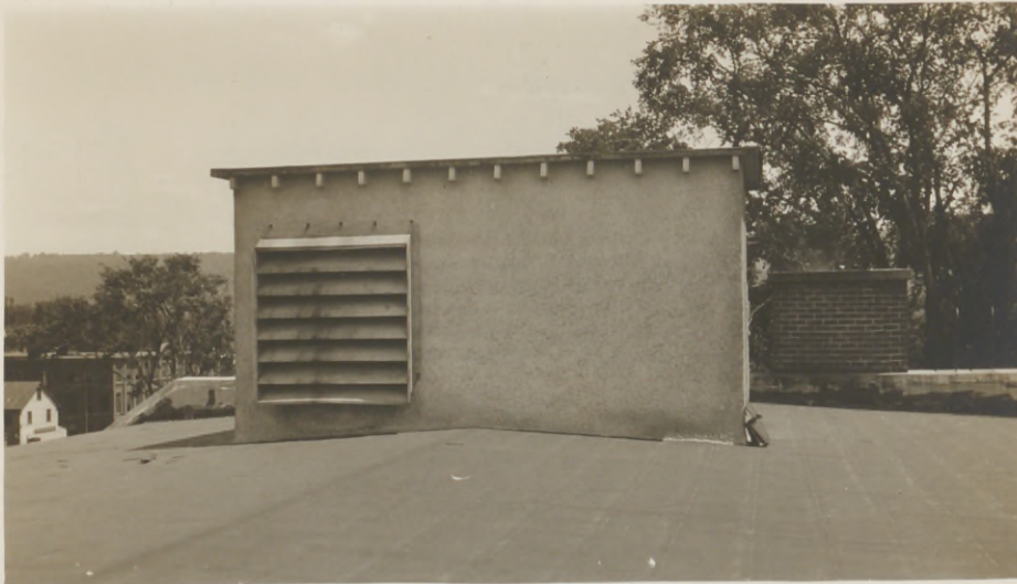
Ventilator on Colonial Theatre
