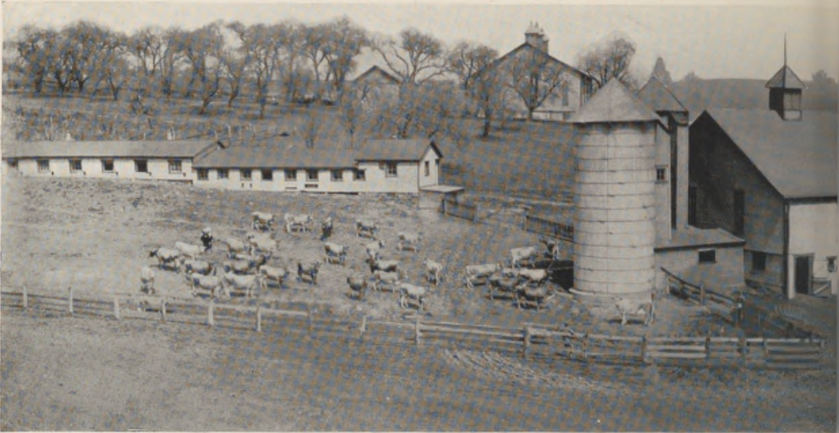
View of Highland Farms Dairy Buildings
