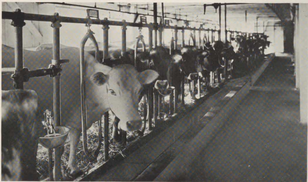
Interior View of Highland Farms Dairy Barn, Showing Stanchions and Individual Drinking Cups, Providing Fresh Water for Each Cow. The Floors are of Concrete
