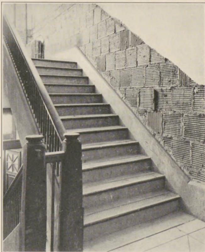
FIG. 22.—Construction of reinforced concrete stairway.
