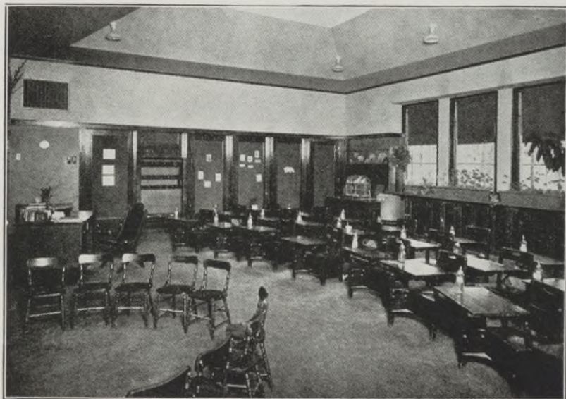
Cook County Winnetka. Hubbard Woods School. Classroom.
