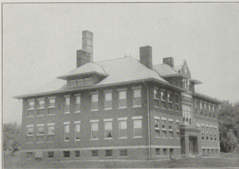
Woodford County. Roanoke. Elementary School. Built 1910. Cost $20,000. Eleven classrooms.
