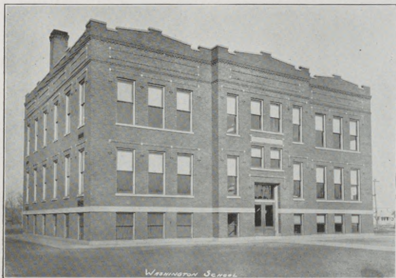
Madison County. Wood River. Washington School. Built 1916. Cost $38,000. Eight classrooms. Gymnasium.
