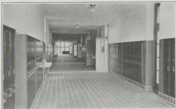
Showing North Corridor with Lockers Recessed into the Walls.
