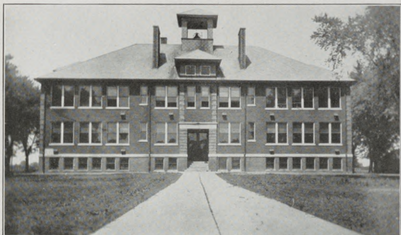
Washington County. Ashley. Elementary and High School. Built 1913 Cost $39,000. Nine classrooms. Auditorium.
