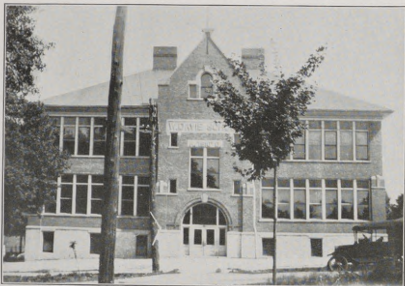
Union County. Anna. Davie School. Built 1910. Cost $20,000. Eight classrooms.
