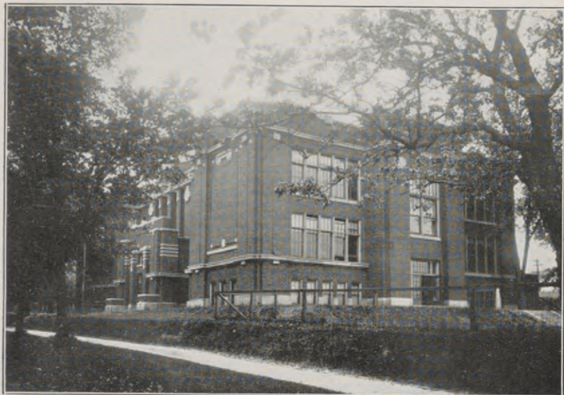
Adams County. Quincy. Dewey School. Built 1918 Cost $94,785. Nine classrooms. Auditorium. Gymnasium.
