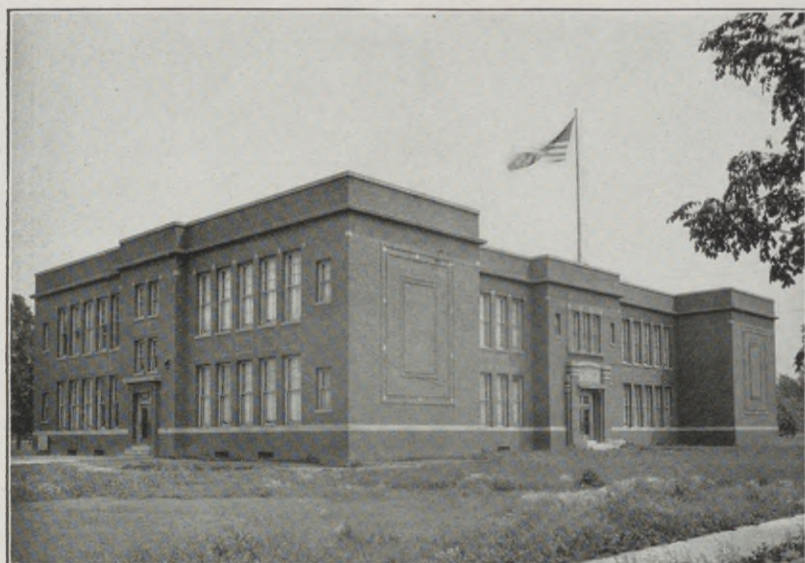
LaSalle County. Streator. Sherman School. Built 1917. Cost $70,000. Twelve classrooms. Auditorium and gymnasium combined.
