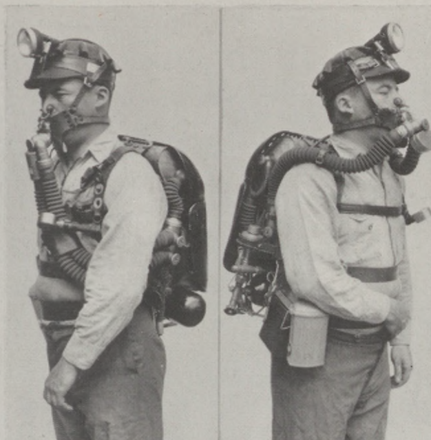
Draeger (1924) 2-Hour Apparatus (with side tubes and shoulder tubes), BM-1304
