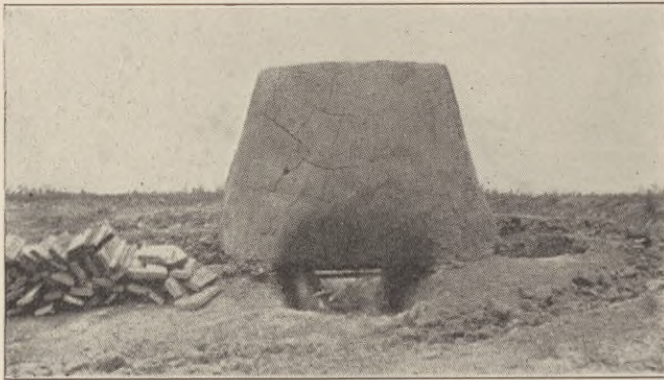
Fig. 33. Barrel and trench incinerator. Barrel made from packed clay moulded over wooden barrel. (From Dunham's Military Preventive Medicine, 3rd Edition).
