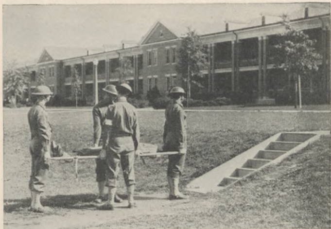
FIGURE 100.—Upstairs carry, second step.
