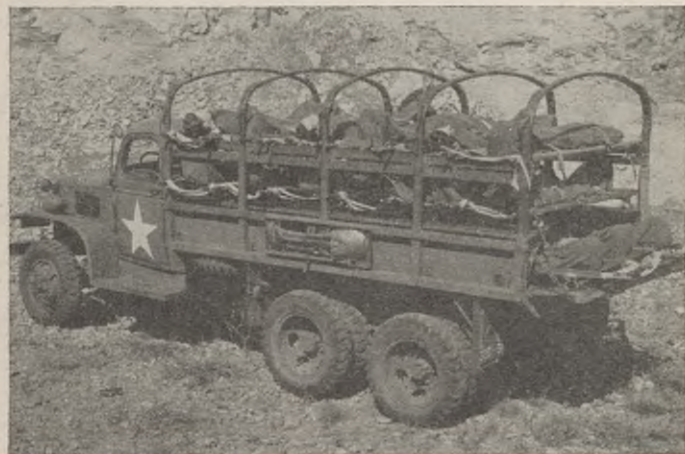
FIGURE 170.—2½-ton truck loaded with eighteen litters.
