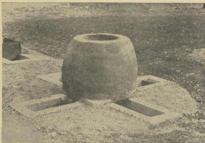
Plate 9. Cross Trench Incinerator with Barrel Made of Packed Clay Molded Over a Wooden Barrel.
