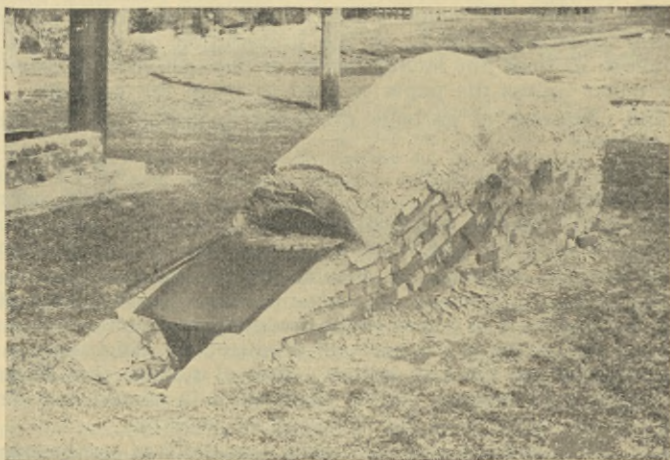
Plate 3. Incline Plane Incinerator.
