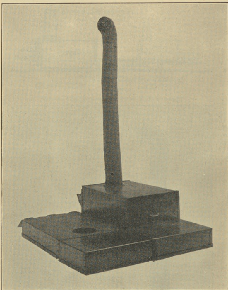
Plate 6. Field range no. 1, set up, rear and right side, with boiling plate and Alamo attachments.
