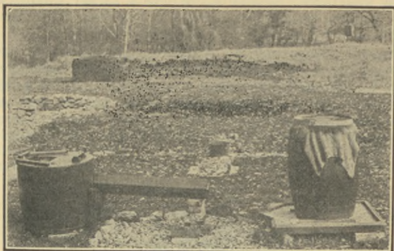
Plate 16. Soakage Pit and Grease Traps. Left, Cold Water Grease Trap; Right, Ash Barrel Grease Trap.
