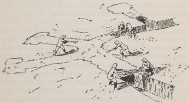
Figure 30. Lattice and snow-covered trenches.
