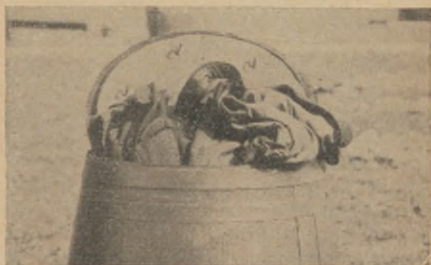
FIGURE 54.—Hooks for suspending material in Serbian barrel.
