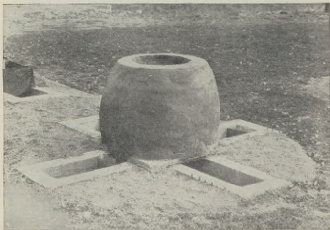
FIGURE 23.—Cross trench incinerator with barrel made of packed clay molded over a wooden barrel.
