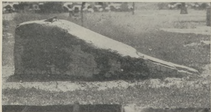
FIGURE 18.—Incline plane incinerator, side view.
