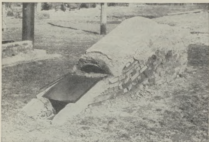
FIGURE 17.—Incline plane incinerator.
