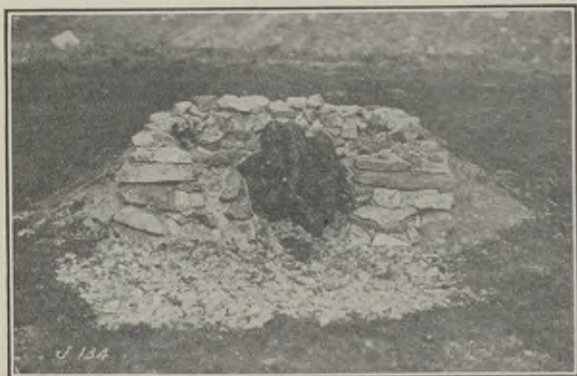
FIGURE 25.—Straub rock pit incinerator.
