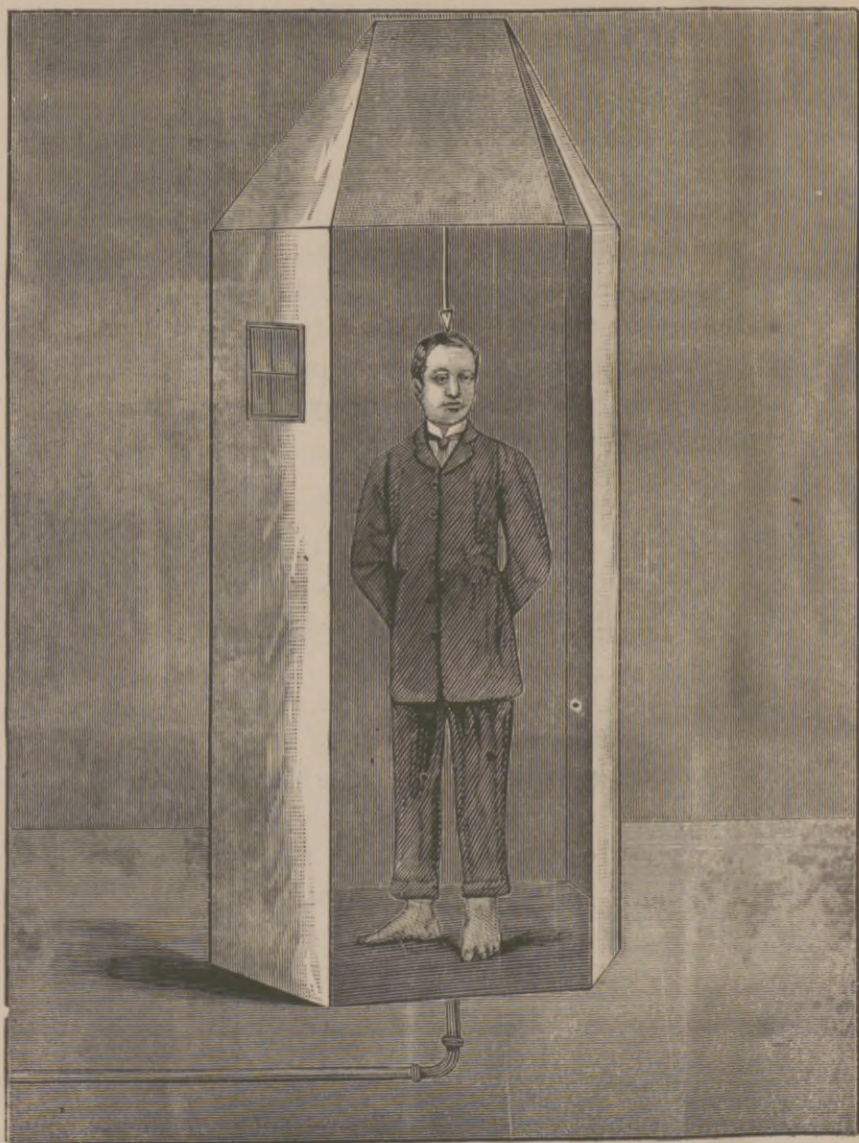
EXECUTION BY ELECTRICITY.
