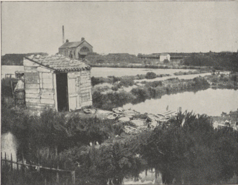
FIG. 2. SABLES D'OLONNE. A VIEW OF THE CLAIRES TAKEN FROM THE MARGIN OF THE GREAT BASIN, SHOWING THE HEIGHT, WIDTH, AND CHARACTER OF THE EARTHEN BANKS THAT FORM THEIR OUTLINES. (Page 378.)
