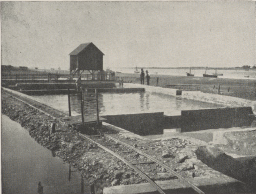
FIG. 2. MARENNES (LA TREMBLADE). A BASIN OF DÉGORGEMENT, CONCRETED, DRAINED BY COMPARTMENTS.
