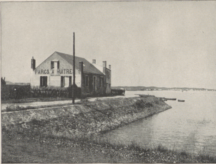
FIG. 1. SABLES D'OLONNE. VIEW OF GREAT BASIN OF ÉLEVAGE TAKEN FROM NEAR THE SLUICE GATE.
