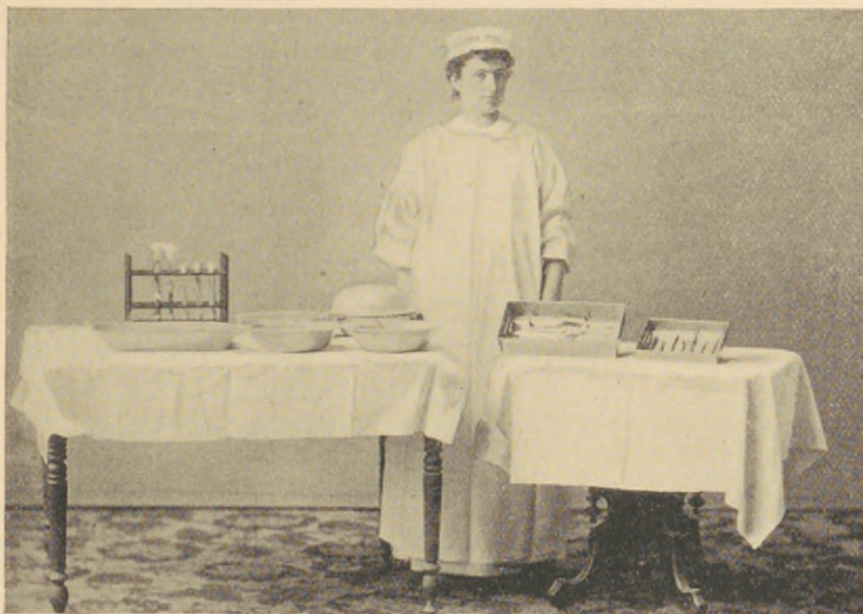
FIG. 6.—Pans, basins, and trays arranged for the operation.
