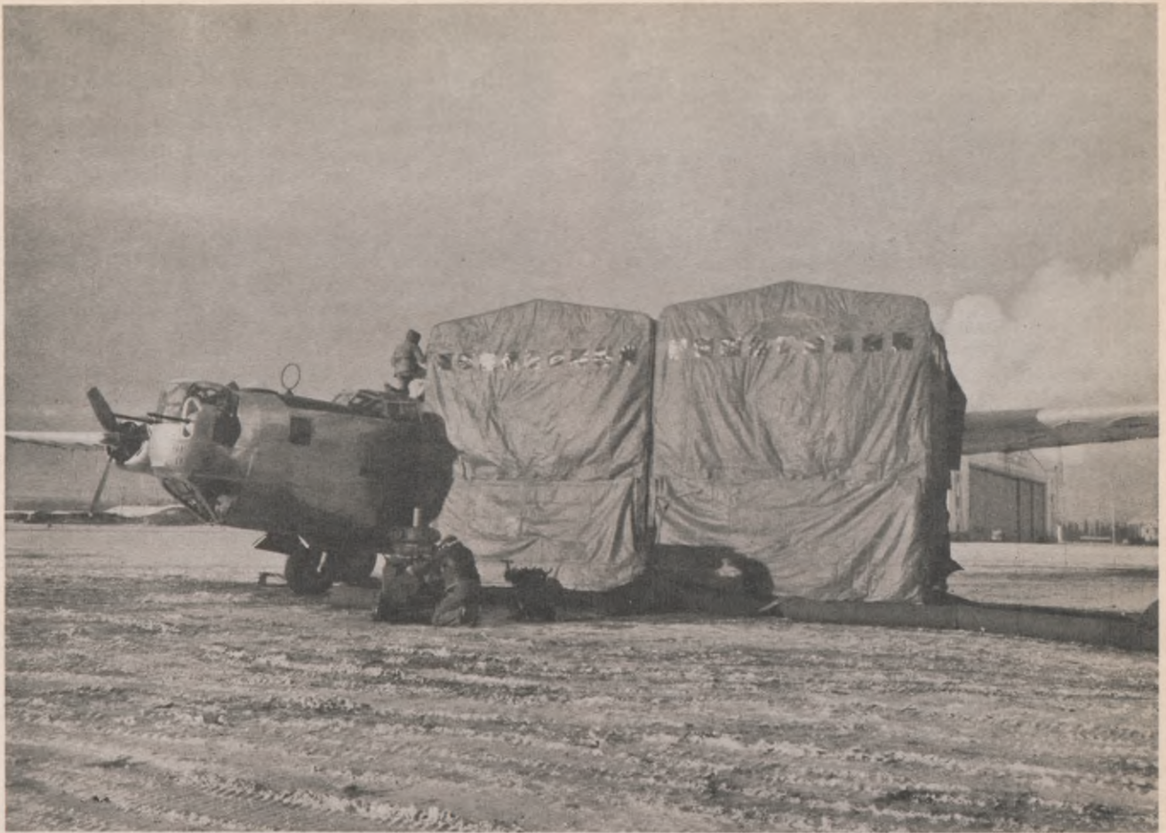
Maintenance using heated nose hangars
