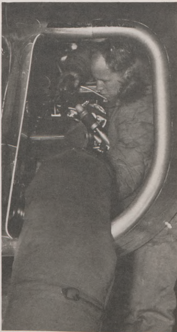
P-59A turbine check-heater duct in use
