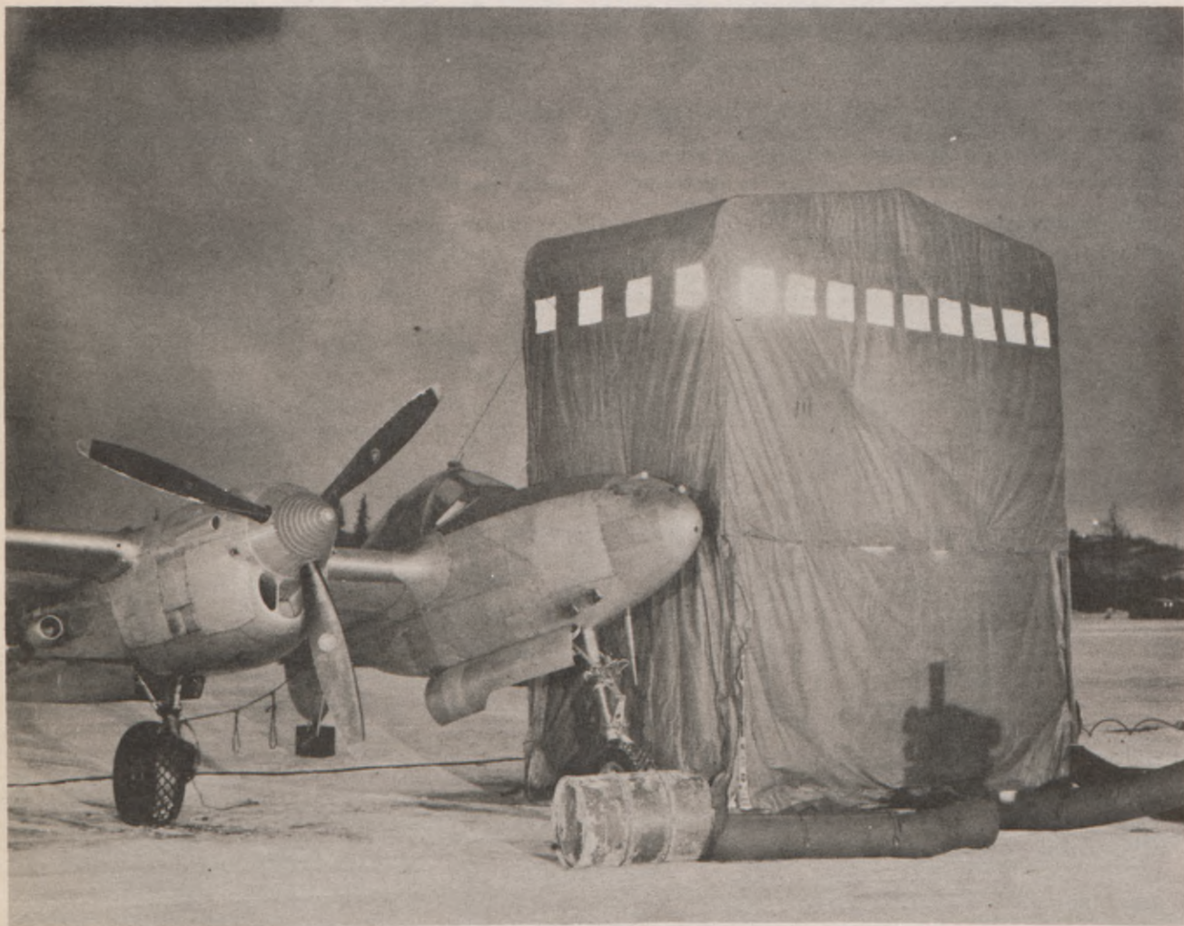
Maintenance Using Heated Nose Hangar
