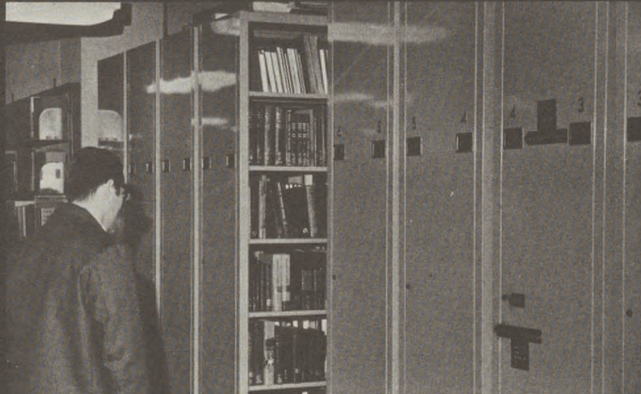
23. ELECTROCOMPACT STACK. AMERICAN UNIV. WASHINGTON D.C.
