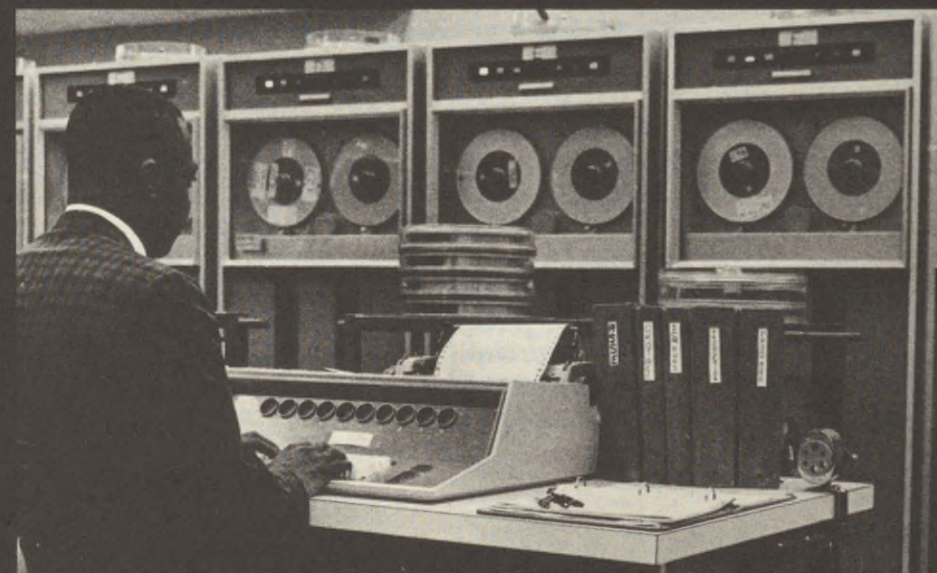
9. MEDLARS INSTALLATION - CONSOLE & PAPER TAPE READERS
