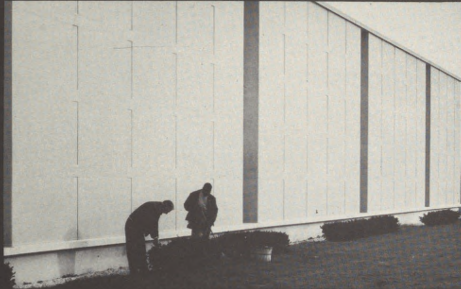
31. EXTERIOR, SHOWING WATER TABLE
