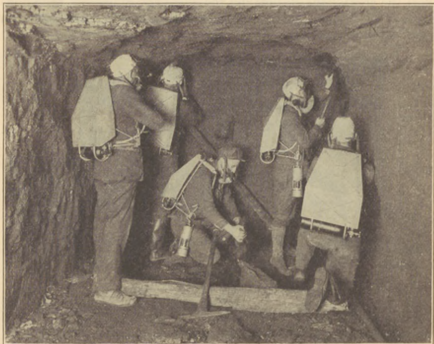
Miners at work underground wearing oxygen breathing apparatus.
