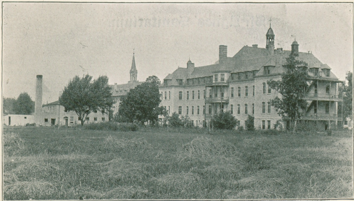
REAR VIEW LOOKING WEST.
