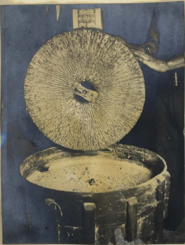
A flour mill in the Polish colony in Sao Matheus, made from a single log cut in two and the two opposing surfaces filled with steel nails.
