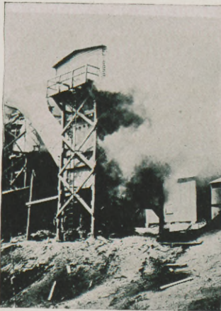
Elimination of Dust or Smoke by Cottrell Process Current off
