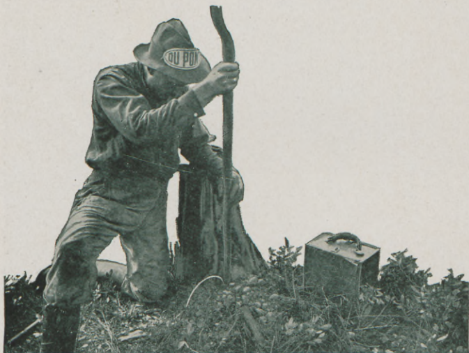
Removing Stumps by Explosives—Tamping the Charge
