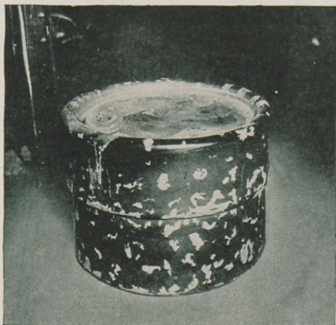
Pot of Optical Glass After Cooling Several Days
