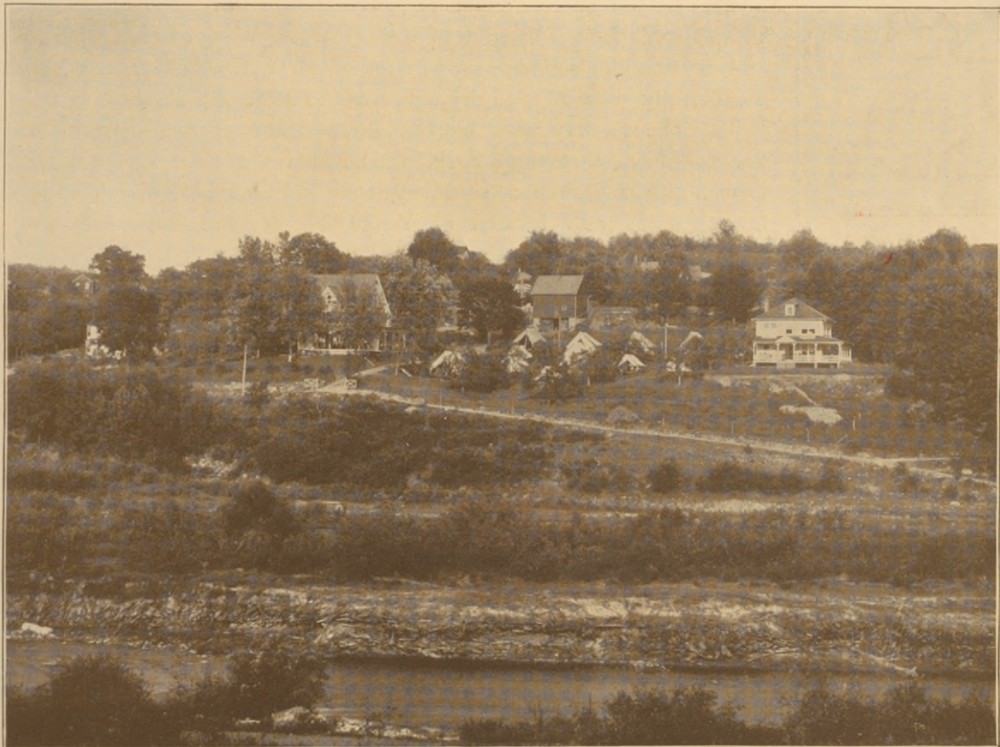
A VIEW FROM THE SOUTHWEST
