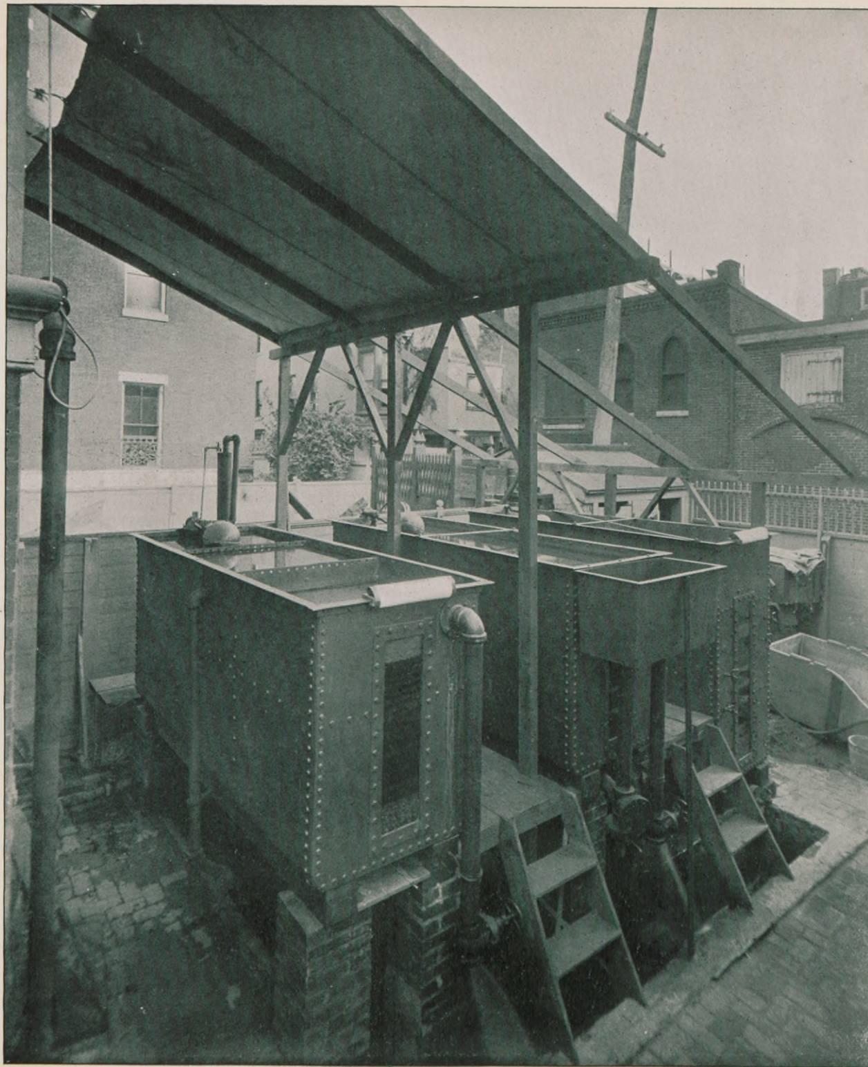
Figure 6. Maignen's Improved Sand Filtration Experimental Plant. 1310 Arch St., Philadelphia.
