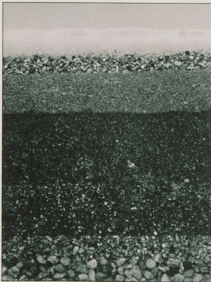
Figure 8. Maignen's Asbestos Felt Membrane on Sand Bed.
