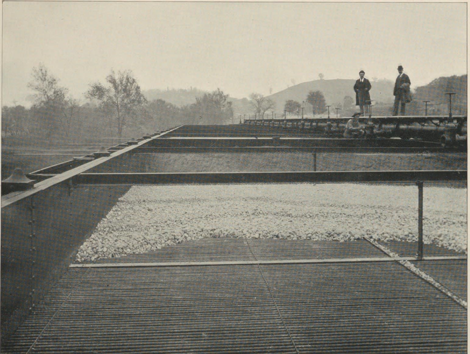
VIEW SHOWING FORMATION OF THE ELEVATED FILTER BEDS LOCATED IN AND OVER RESERVOIRS.
