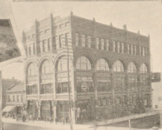
NEW DAILY BUILDING
