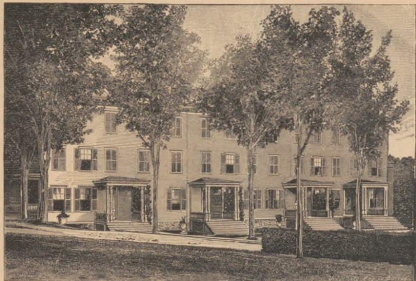
The Pavilion—Cottage Building and Cottage Flats D, E, F, G.
