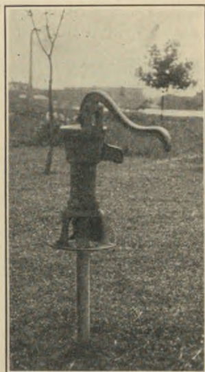
A DRIVEN WELL Nothing can fall into it.
