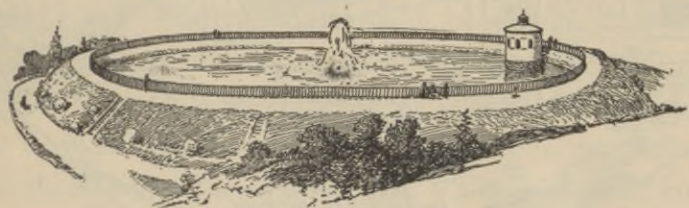
RESERVOIR FENCED IN FOR PROTECTION.
