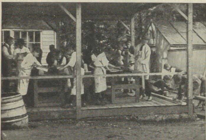
FIG. 98. In this outdoor school in London, England, the boys are building their own schoolhouse. The pupils were sent to this school because their health was poor and they needed outdoor life and fresh air. (Courtesy of Mr. H. Broughton)
