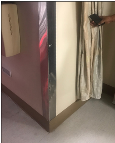
Wall corner with metal protective cover
