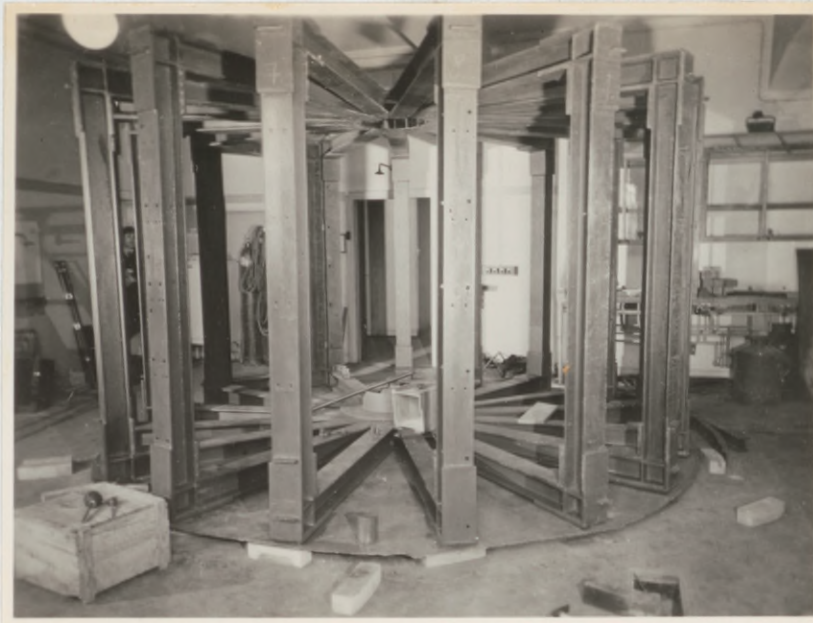
Above, the low pressure chamber is shown being installed at the Aero Medical Center. It was moved to Heidelberg from the Munich Institute for Aviation Medicine at Freising.
