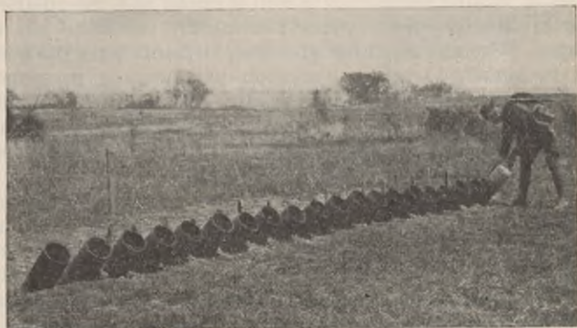
FIGURE 2.—Installed chemical projector battery.
