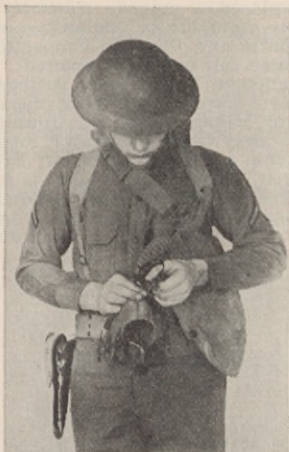
FIGURE 37.—INSPECT MASK. TWO. Examining outlet valve.
