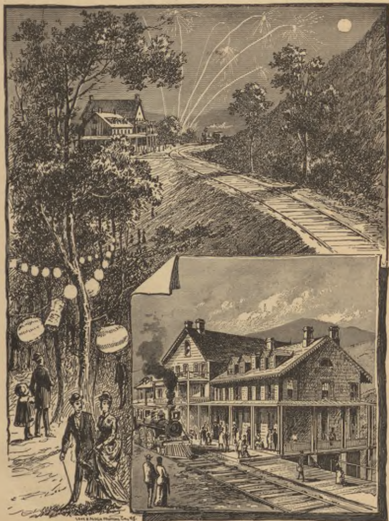
THE MAIN HOTEL—MORNING AND NIGHT.
